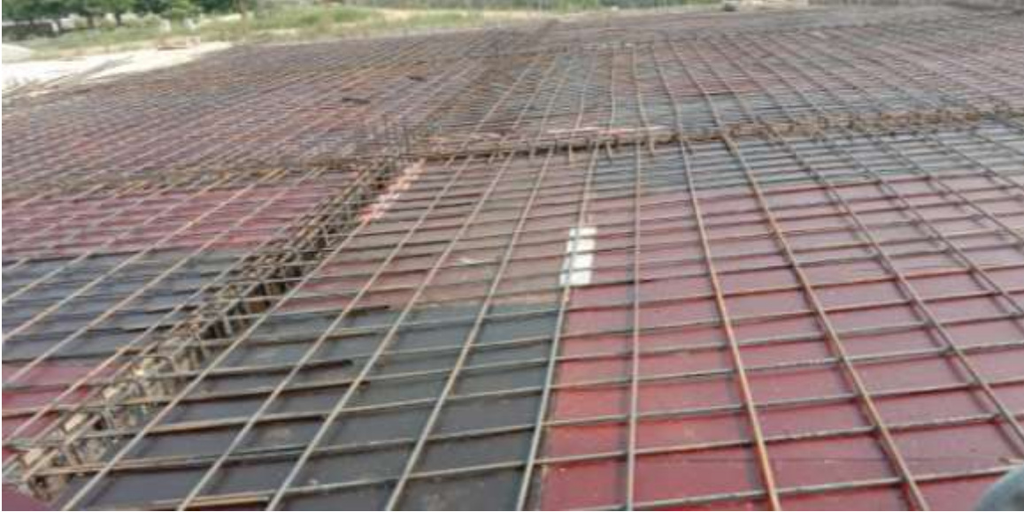
Picture 3: Steel Fixing of ABR Slab
