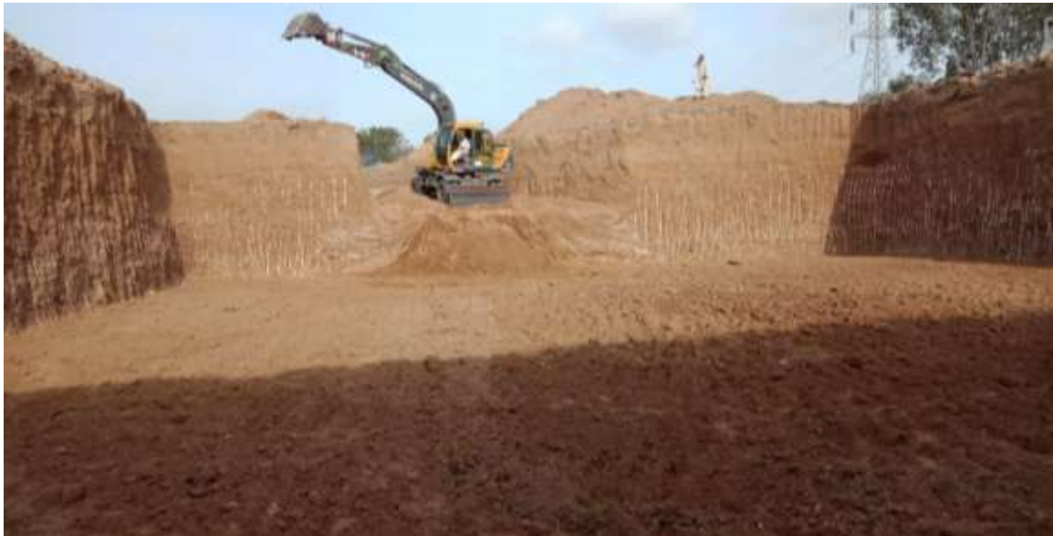
Picture 2: Excavation of ABR Tank
