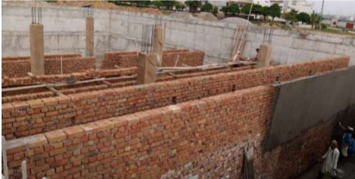
Picture 1: Construction of Partition Walls in ABR Tank
