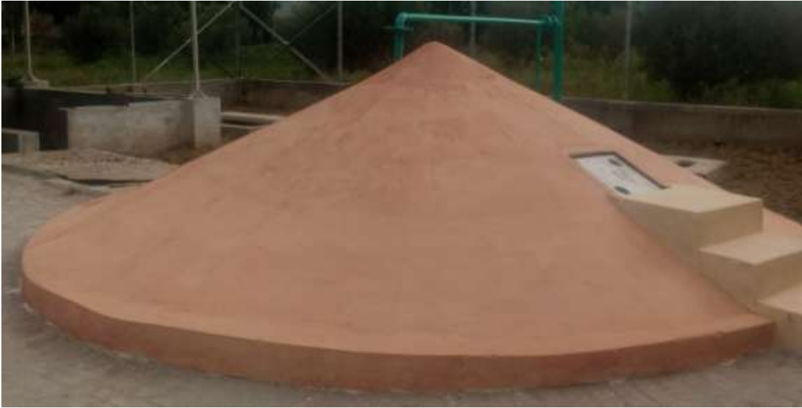
Picture 3: Bio-Digester Tank
