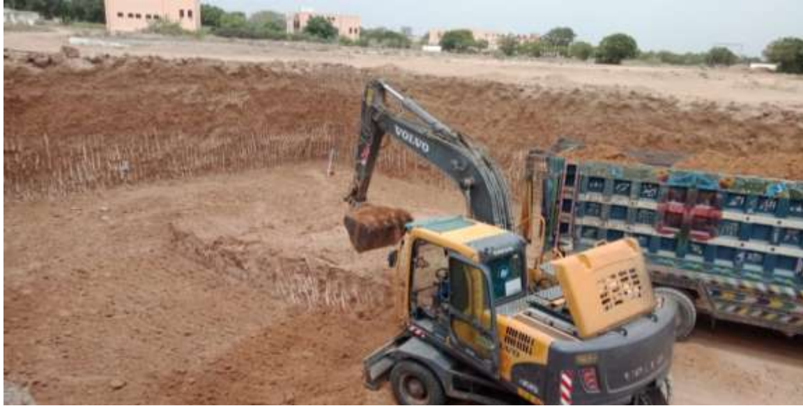
Picture 1: Excavation of ABR Tank
