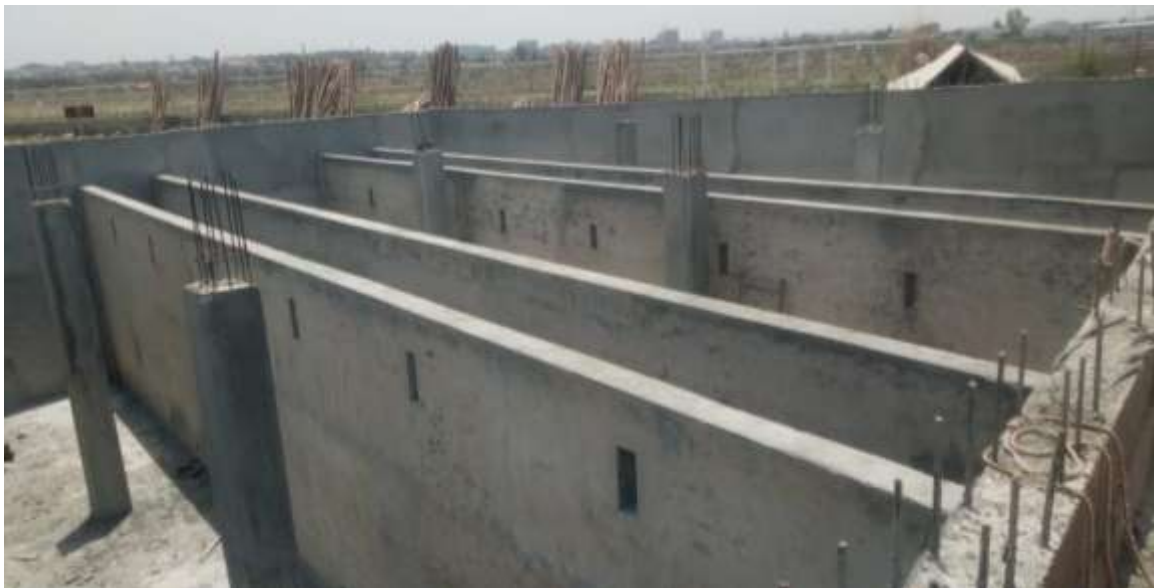
Picture 2: Plaster of Partition Walls in ABR Tank
