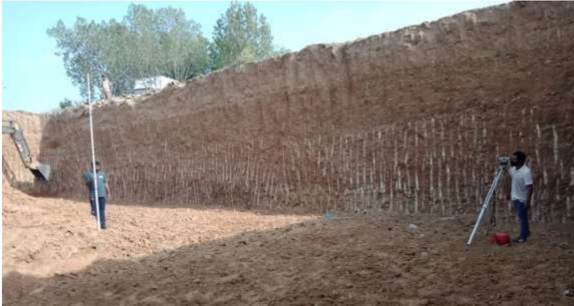
Picture 3: Excavation Level Checking
