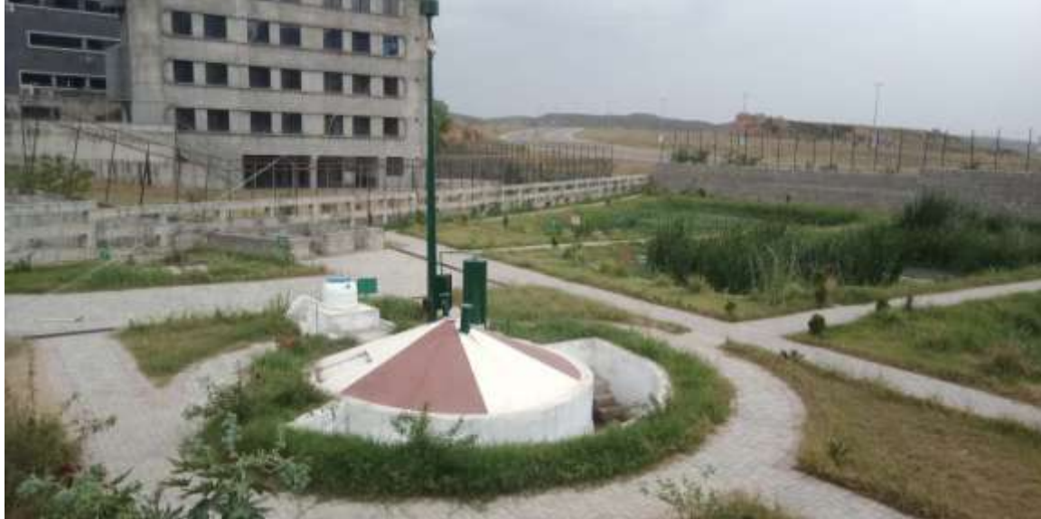
Picture 1: Overview of STP
