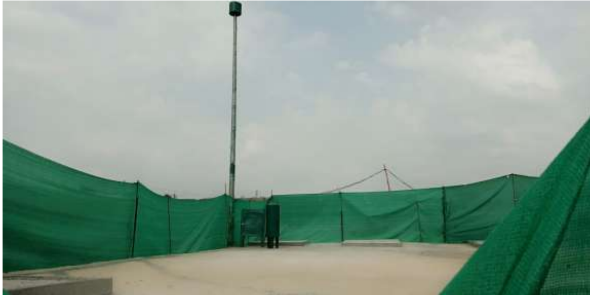
Picture 1: ABR and Bio gas incinerator
