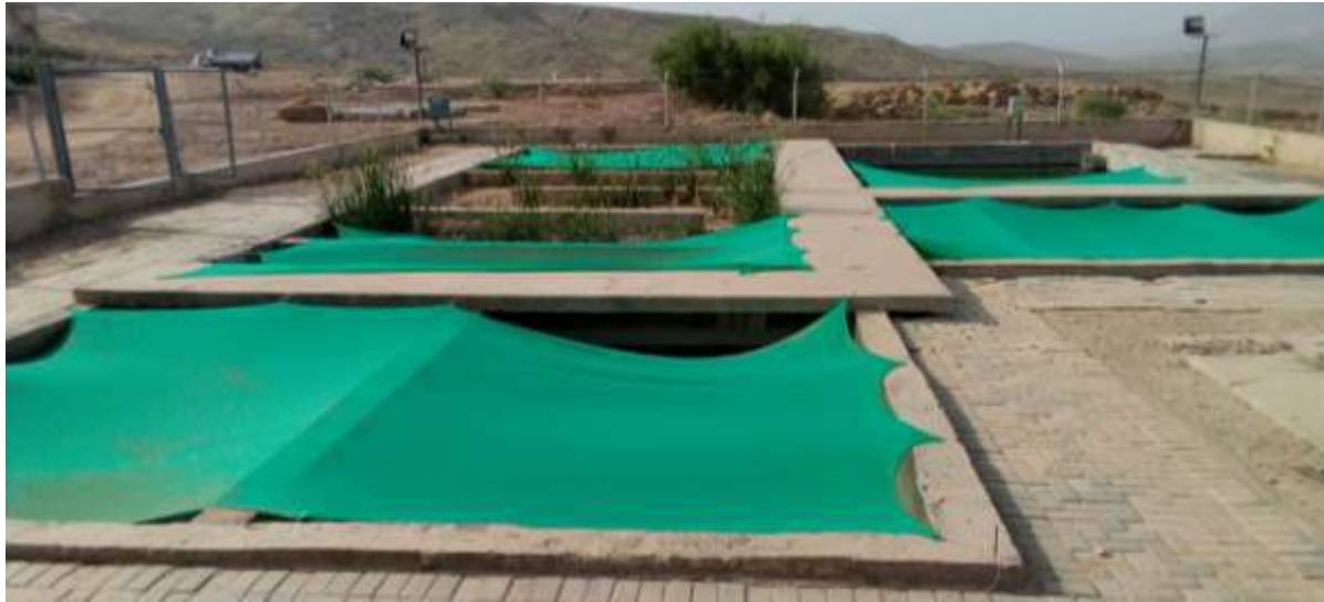
Picture 1: Overview of STP
