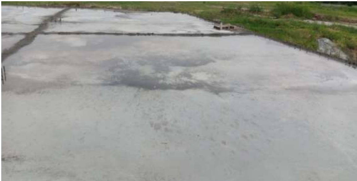
Picture 4: Slab on ABR Tank
