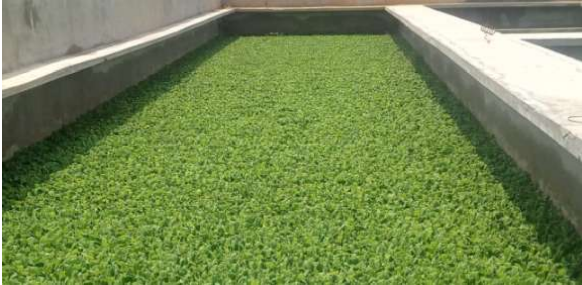
Picture 3: Treated Water Pond
