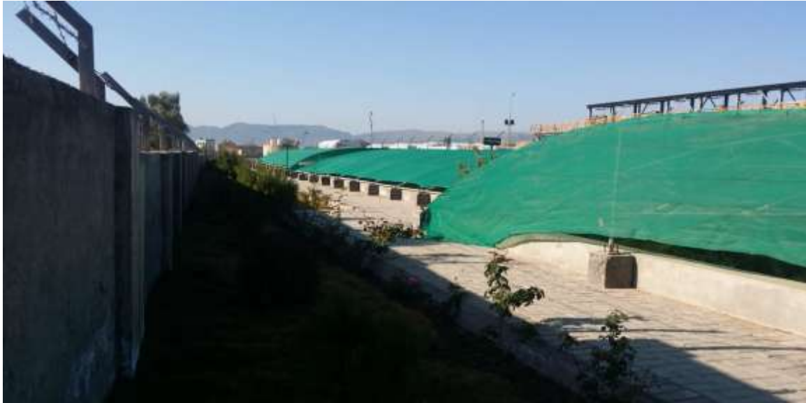
Picture 2: Phytoremediation, Sand Filter Pond and Treated pond
