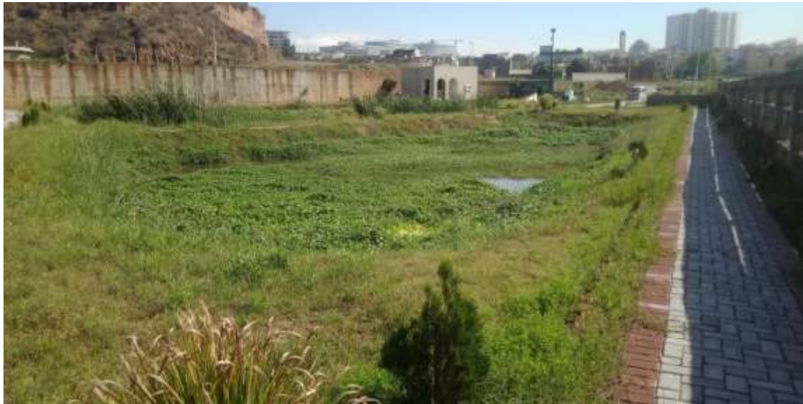
Picture 3: Treated Water Pond
