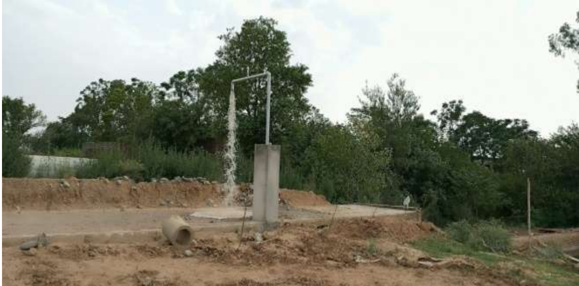
Picture 3: Treated Water Filling Station Point
