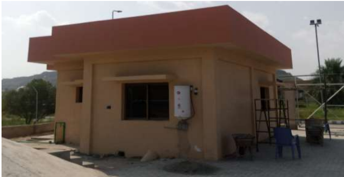
Picture 1: Collection + Segregation Hall
