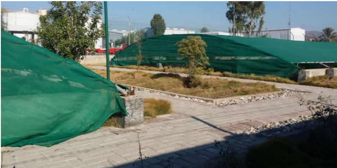
Picture 2: Sedimentation and Wetland Pond
