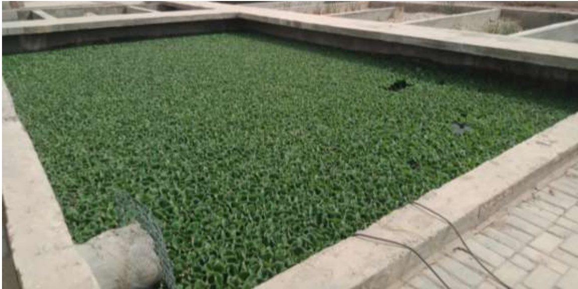
Picture 3: Treated Water Pond
