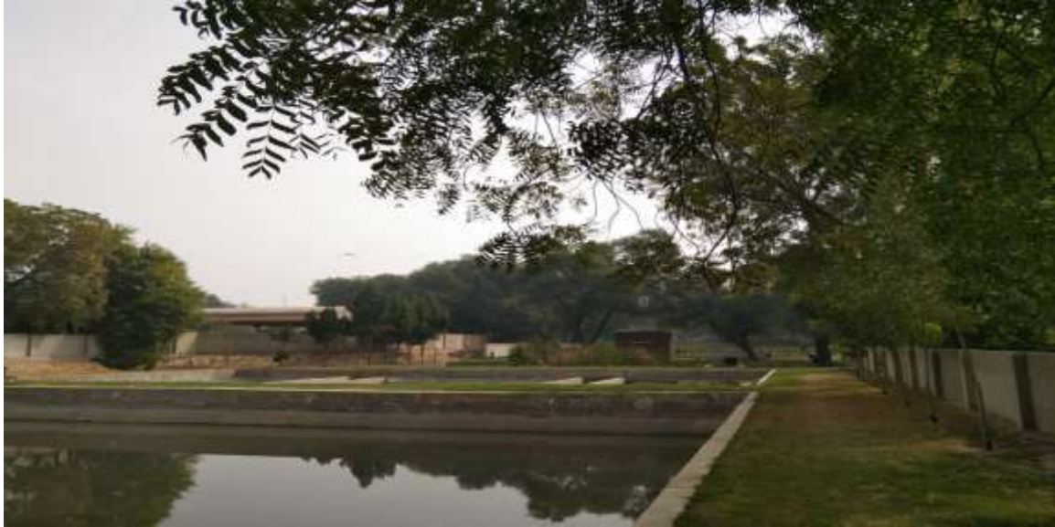
Picture 3: Treated Water Pond
